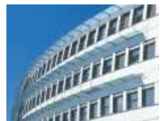
ENERGON Ulm: The administration building of the Software AG foundation is the largest office building in the world built to the passive house standard. Thermix® warm-edge spacers are built into the windows and the facade.
